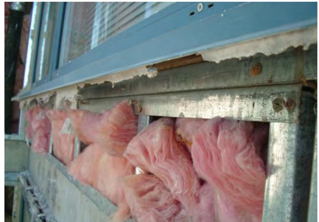
*Corroded screws in stud wall beneath window*
